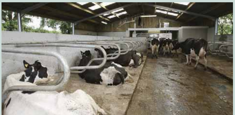
Well-designed sheds are easier to muck out, clean down and bed up, meaning that these essential operations are carried out more often and more effectively
