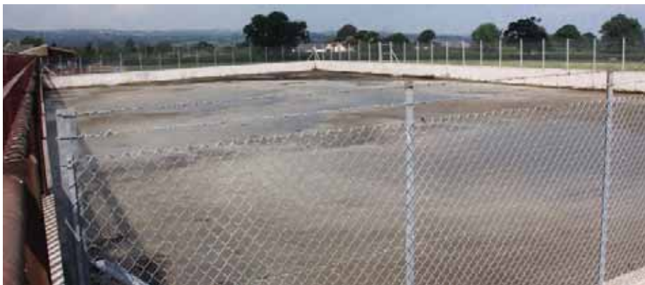
The new slurry store at Bryn Mawr Farm can hold five months' worth of slurry and has resulted in reduced fertiliser usage and significant labour savings.
